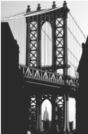
The Empire State Building seen through the arch of the Manhattan Bridge.
